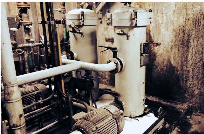
The SAG Mill's two 16" diameter canister filters.
